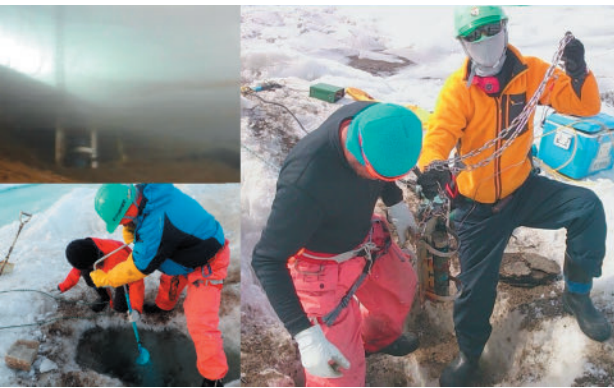
Photo 5. Underwater tide gauge (upper left), ice drilling (lower left), and tide gauge recovery (right) in Skallen.
