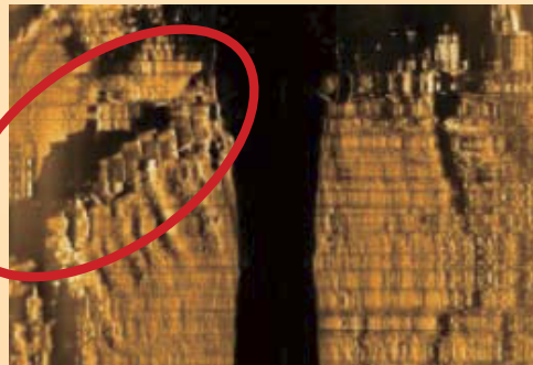
The damaged breakwater at Port of Ofunato
